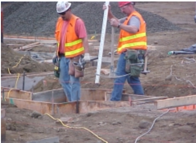
Michael Adcock & Dave Bratlien setting footing forms to grade.
