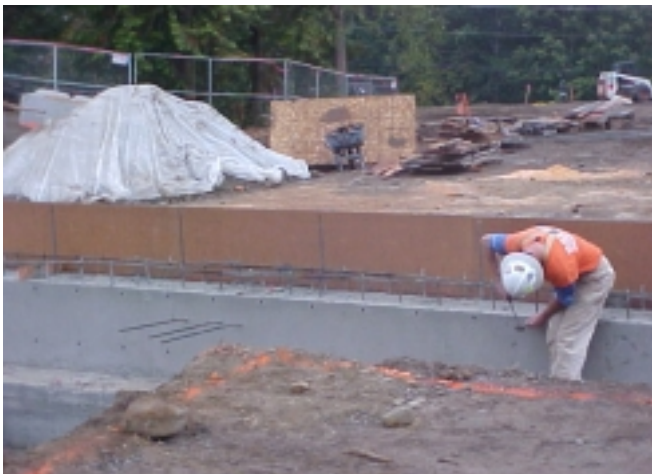
Robert Fischer plugging snap tie holes at boiler room retaining wall.
