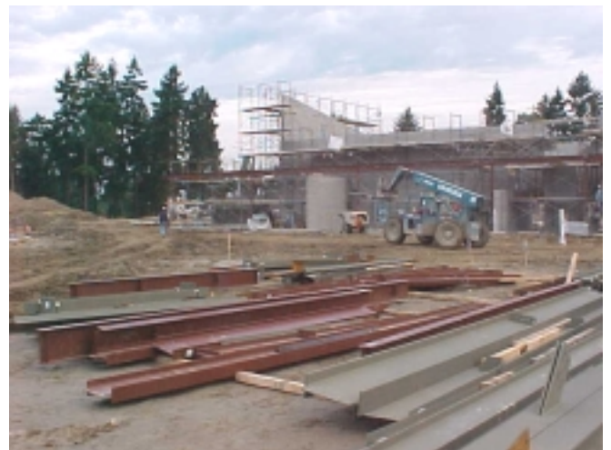
First delivery of structural steel with Activity Wing in the background.
