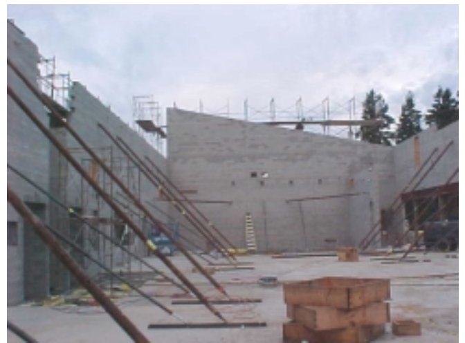
Inside the Activity Wing – topping out CMU walls.
