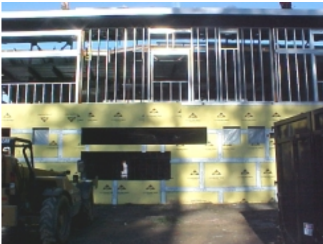
12/15/04 – Dens Board and Metal Framing at SE Wing
