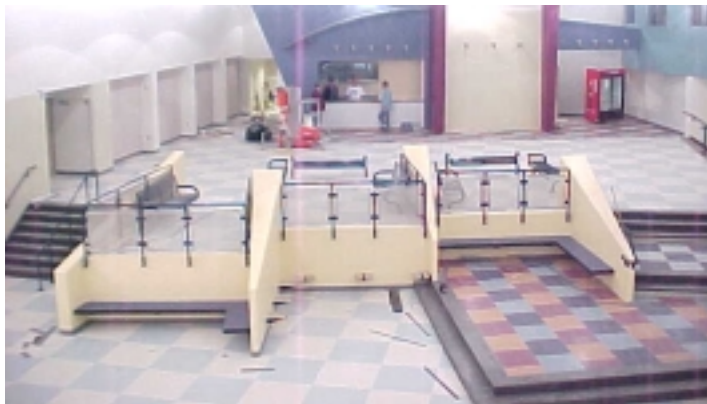
Hazen High School - Commons Area
