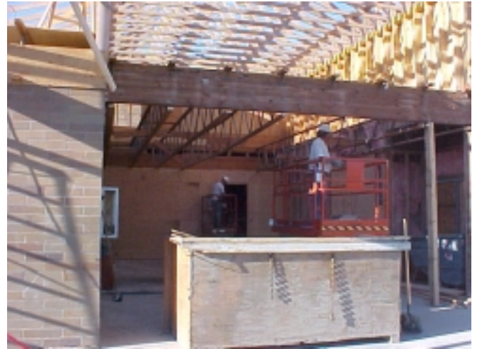
Demo for the Main Entry Well Underway
