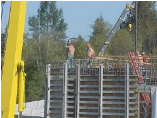
Monte and Mike sting (vibrate) another 90-yard wall pour.
