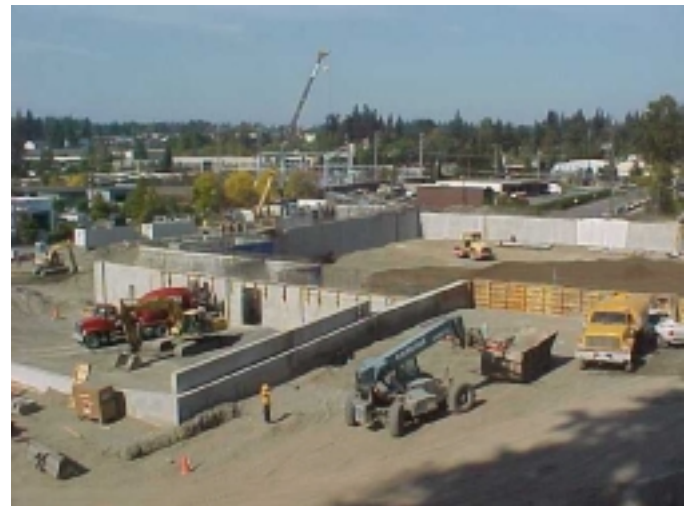
Transfer building pad with part of retaining wall G.
