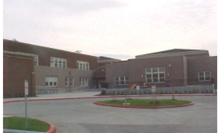
Superintendent: George Mason Sr. Project Mgr.: Steve Hansen Proj. Engineer: Paul Kocharhook Project Manager: Dirk Kilgore
