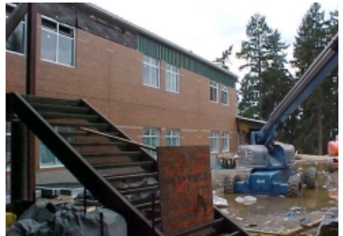
03/25/05 – Typical two story Classroom Wing.
