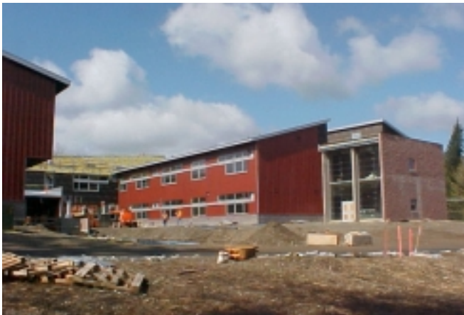
03/30/05 – NE Wing Classrooms with loading dock to the left.
